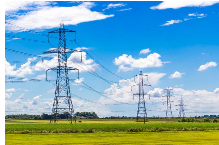
Pylons carry overhead power cables
